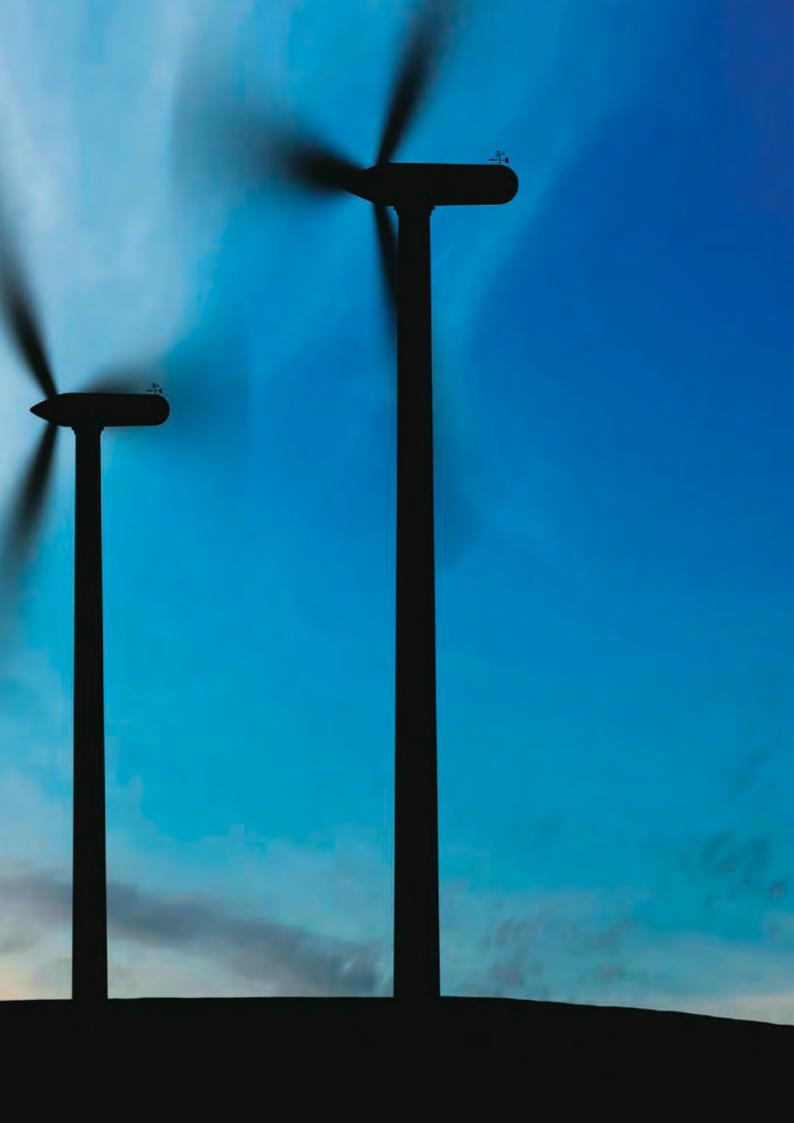
A typical wind turbine on a UK site will be generating for 85% of the year, and on a good site will produce an equivalent of about 30-40% of the electricity that would be produced if you ran the generator at full power by some other means for 100% of the time. On this typical UK site the wind turbine will generate enough energy within 3 months of operation to replace the energy used in making it. Over the course of its 20-25 year life therefore it will repay the energy back some 30 times.
