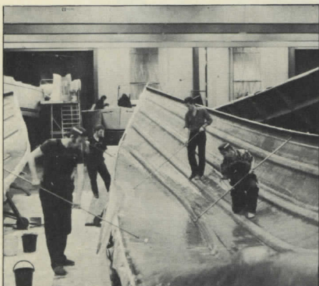
Hand laying of the GRP hull moulding to ensure a perfect finish. At this stage, the mould is still split into its two halves.
