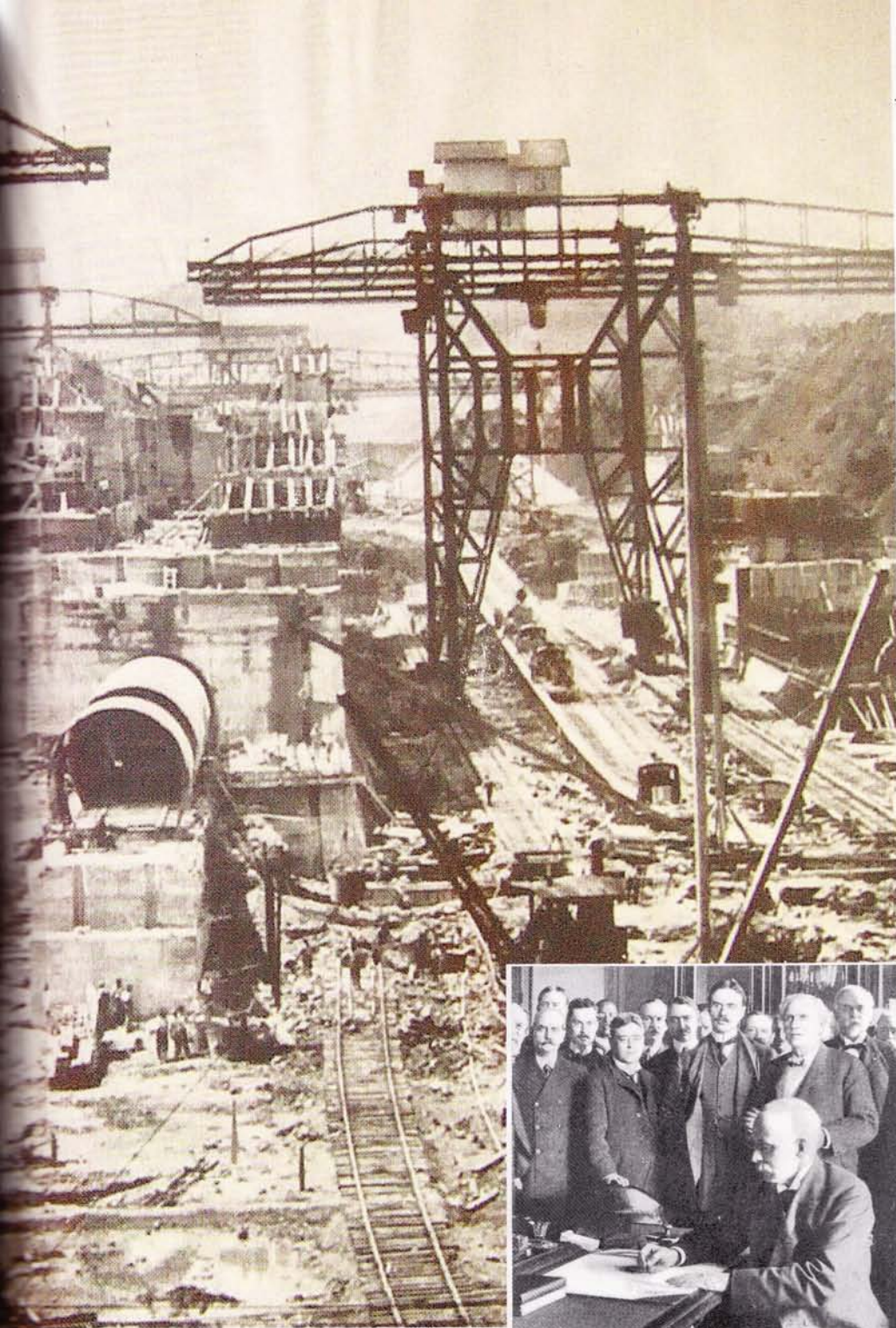
The Gatun flight in construction showing the scale of the locks and culverts. Right: signing the treaty that gave the canal to the US for $40m in 1904
